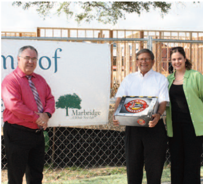
Roxy Van Loo (TIBH), James Stacey (CEO of Marbridge) and Becca McPherson (vice president of development at Marbridge) visit the construction site of Marbridge's new living, office and recreation space, the Lodges."
